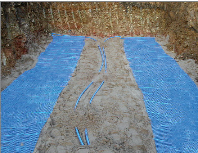
Fig. 78: Installing the compact collector
