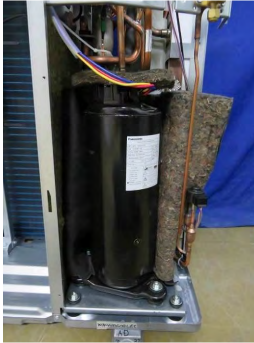
Picture No.7 : Compressor compartment of outdoor unit
