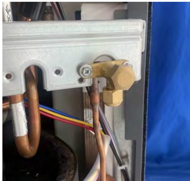
Picture No.8 : Service port compartment of outdoor unit
