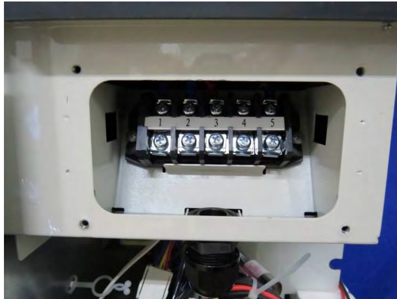
Picture No.5 : Supply terminal of outdoor unit
