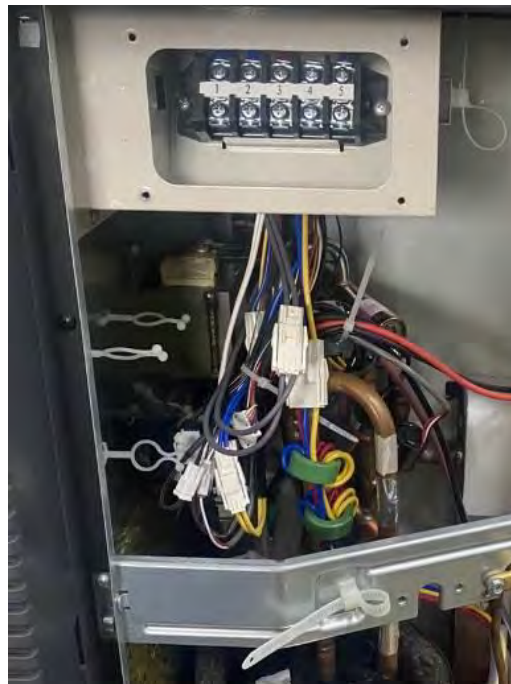
Picture No.6 : Cord anchorage compartment of outdoor unit
