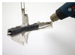
Heat the shrink tube and properly reclose the damaged area.
