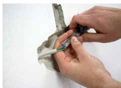
Connect the cable using the cable repair kit.
